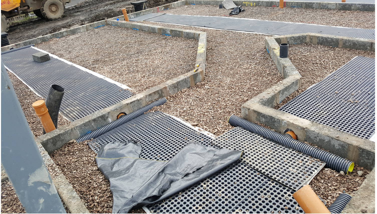
Landflex 25 Gas Venting Geocomposite designed to suit the gas emissions identified in the SI report / verification plan
