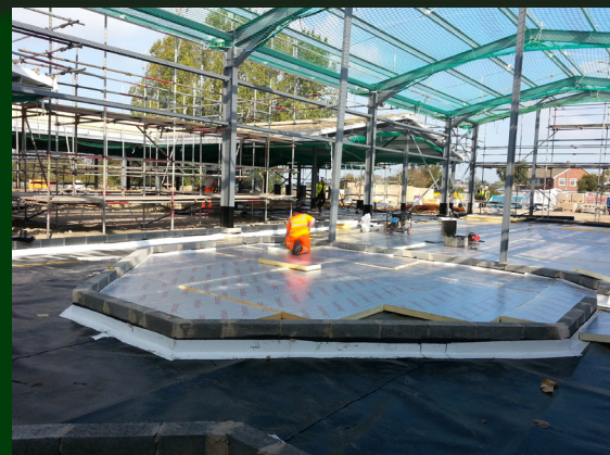
Gas Barrier Installation in a newly built Primary School
