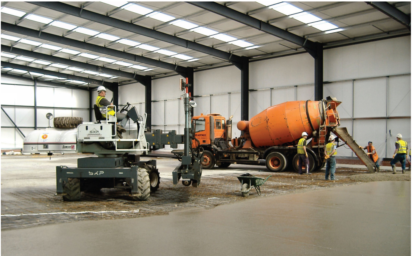
Ridgeons Sudbury, Laser Screeding over PE200HD 2.0mm Landflex HDPE gas membrane
