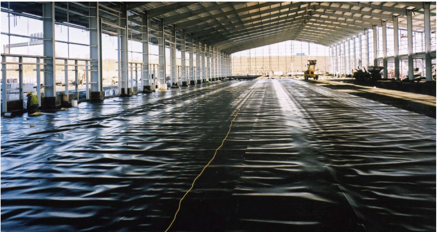
Cambuslang Investment Park, Gas Protection: W A Fairhurst & Interserve
