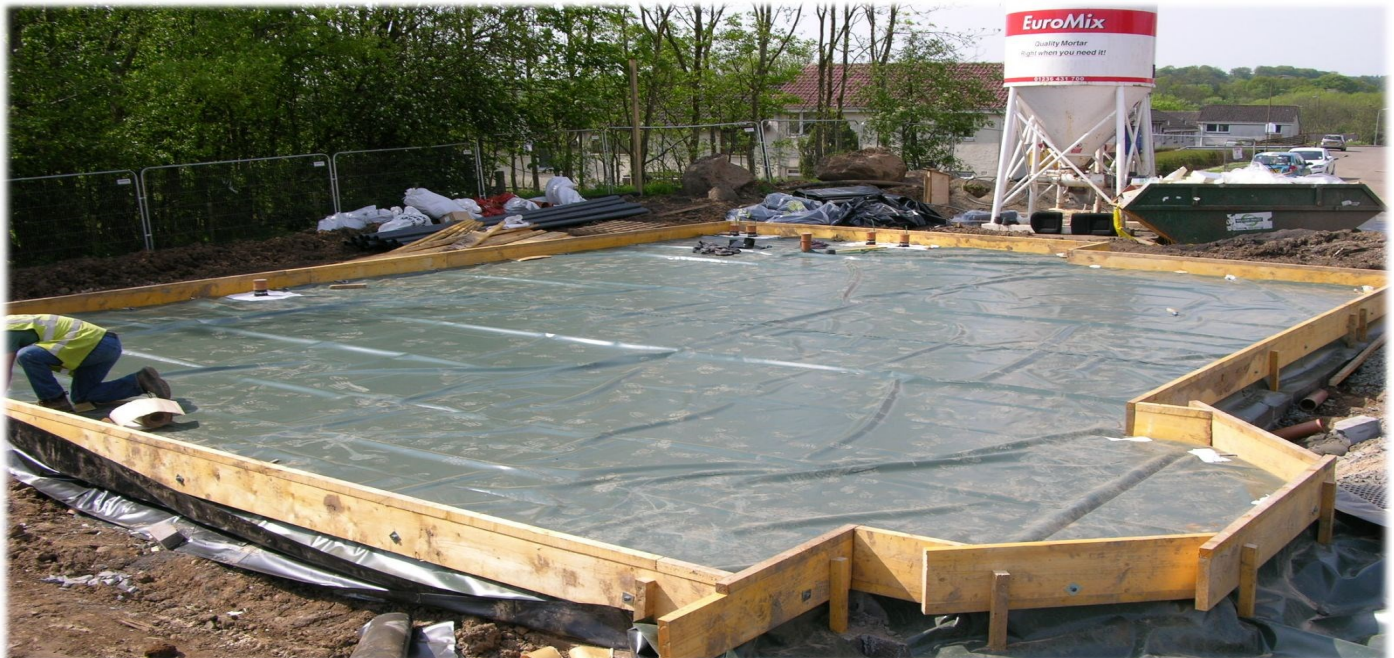
Gas Membrane Supply, Pre Fabrication, and Installation
